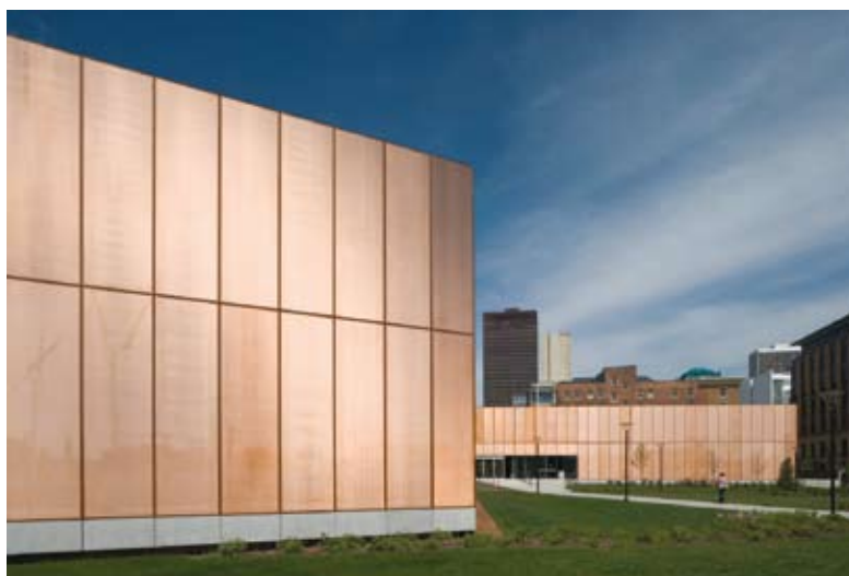
Des Moines Library, USA. Encapsulated expanded metal within glass to achieve this stunning Day/Night effect.
