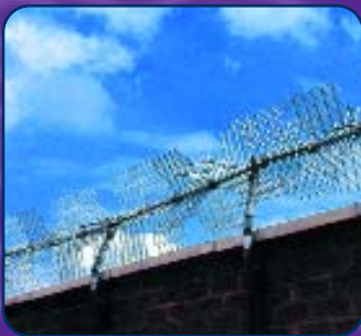
Anti vandal scaling barrier
